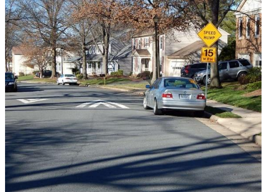
Figure 1: 22-Foot Speed Hump
