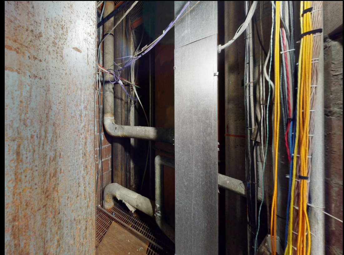
EXISTING SHAFT INTERIOR
