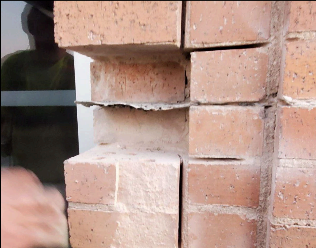
Uncovered Expansion Joint Material
