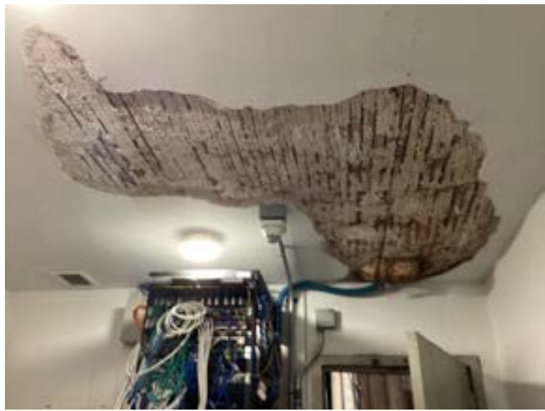
Picture taken at 7 th floor janitor room
