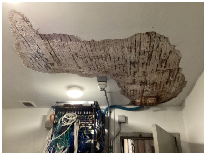
Picture taken at 7 th floor janitor room
